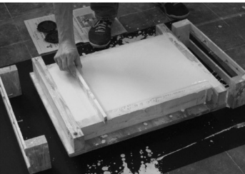
11. Screed top for level surface
